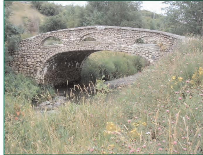
Stone Bridge in Original park section.
