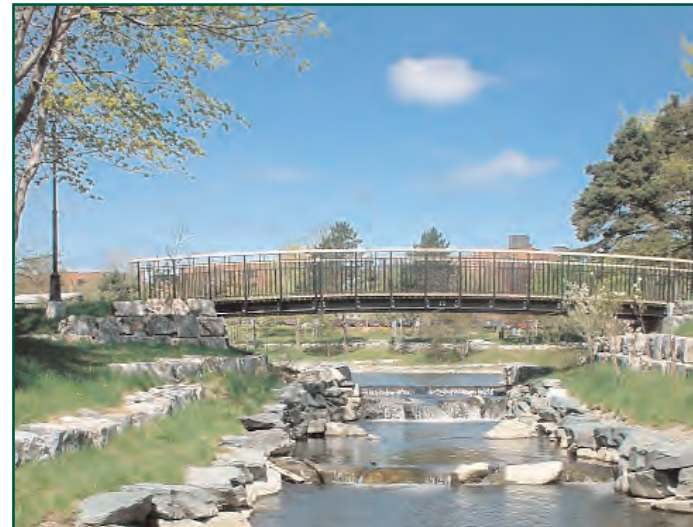
Bridge over the new fish ladder at the Duck Pond.
