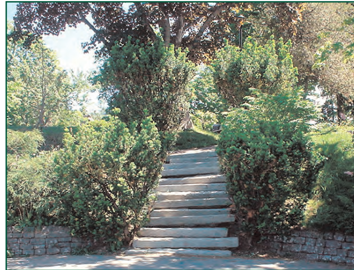
Enhanced maintenance poses a safety issue in areas.
