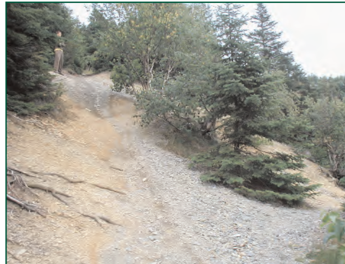
Erosion is a concern raised by Stakeholders.
