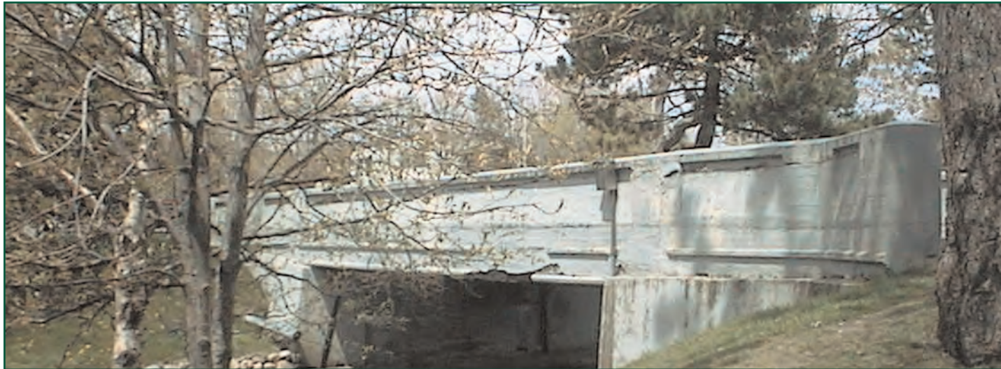
Concrete bridge at the east entrance to the park, 2004.
